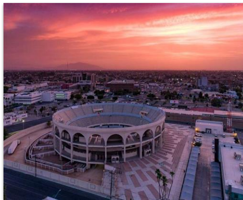
Mexicali, Mexico Average humidity level 55%
